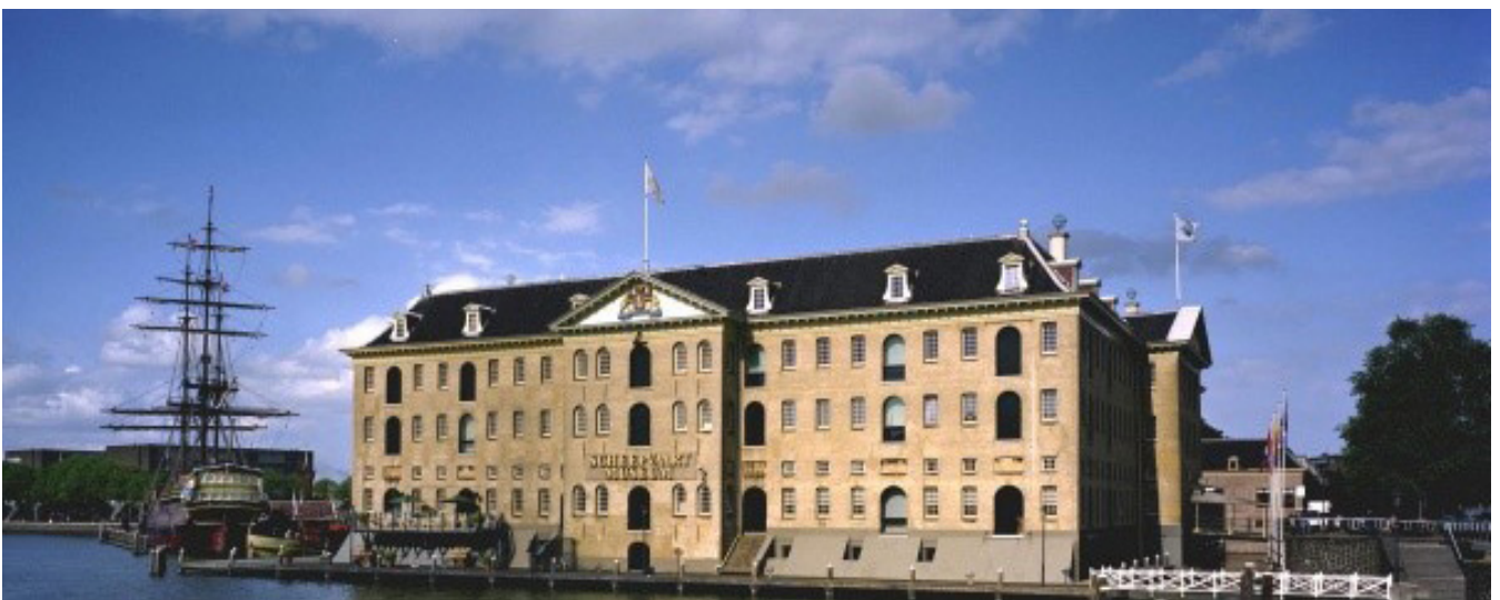
Figure 1: The former warehouse and office of the admiralty, now the Maritime museum. On the background of the conference area.
